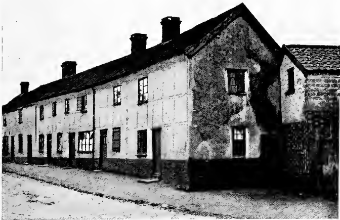
A ROW OF CLAY-LUMP COTTAGES. The front has been plastered and panelled out. In the upper part of the stable building, seen in the foreground, the clay-lumps are shown exposed.
